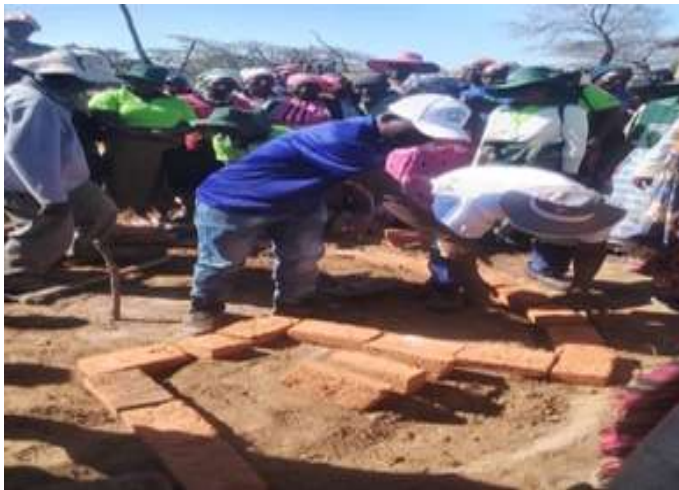
Figure 4. 2: KHG Construction phase 1
