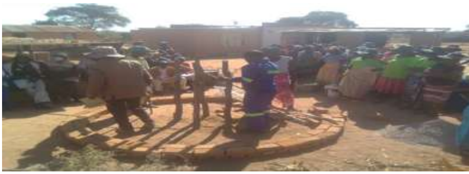
Figure 4. 3: KHG Construction phase 2
