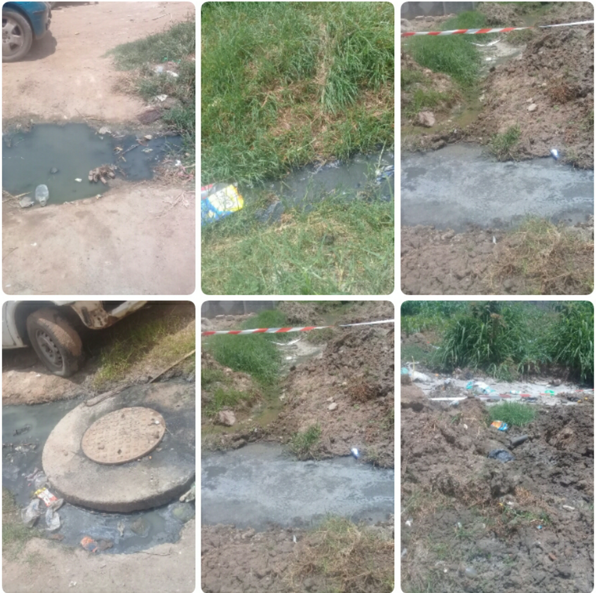
Figure 30: sewer burst and blockages
