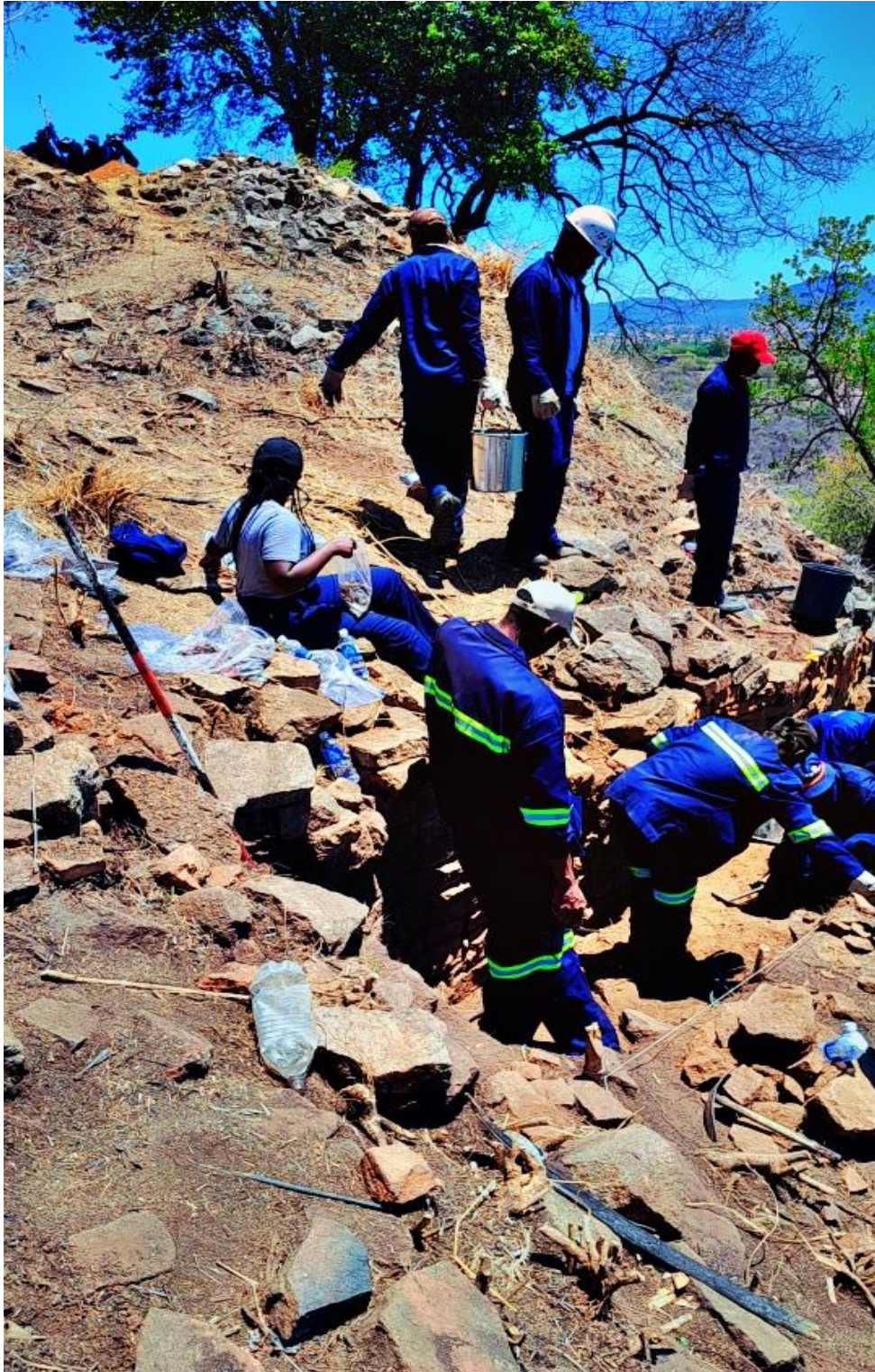
Figure 1: A figure showing excavation being conducted to identify the problem of the wall and to recover buried stones
