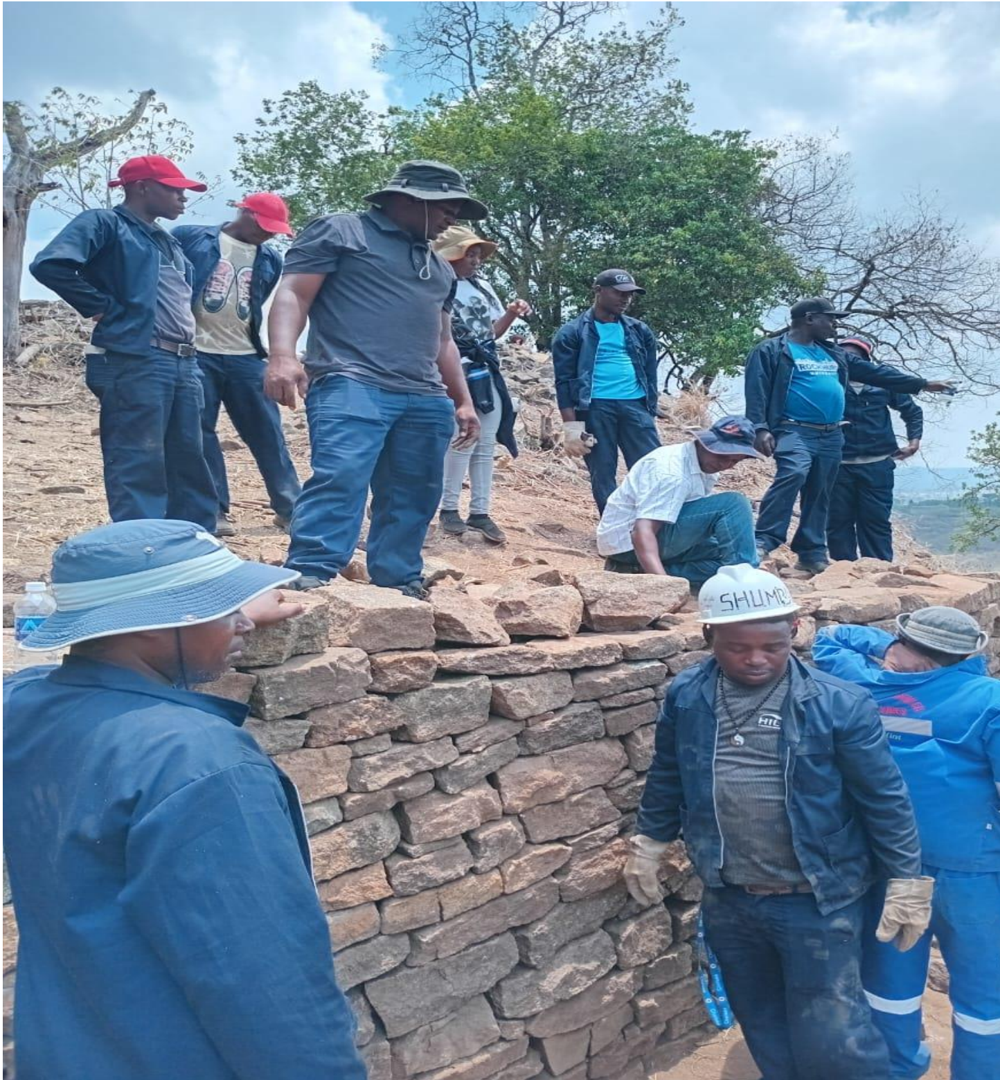
Figure 3: Figure 3 showing the wall after being reconstructed
