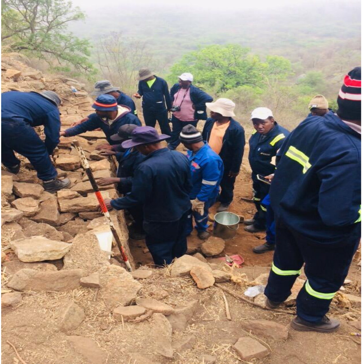
Figure 2: Figure 2 shows stone masons reconstructing the wall using traditional material around the area to fit on top of the wall
