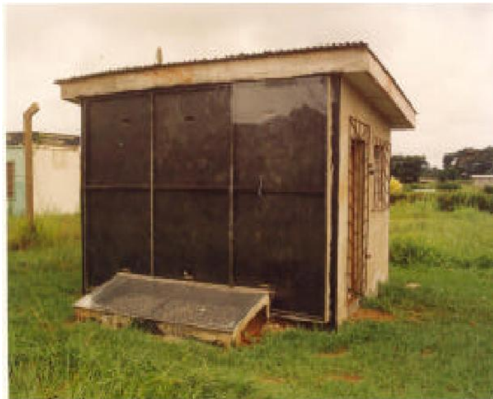
Figure 2.3: Showing the Trombe wall
