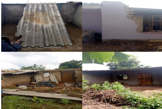
Figure 4.5 Substandard houses that were destroyed by heavy rains during 2022-2023 rainy season (Source: Primary data 2023)
