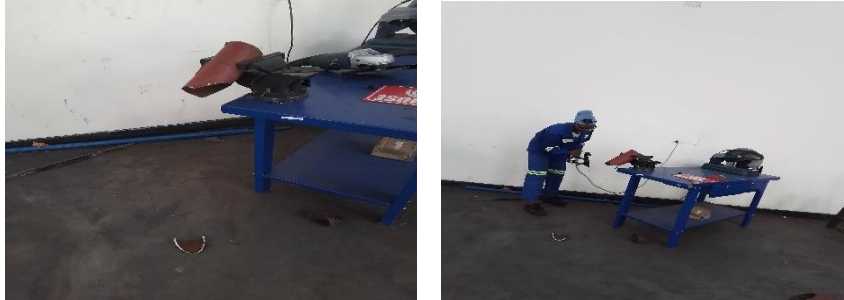
Figure 4.3 : Cutting marked angles on steels whilst clipping the steel on a bench vice
