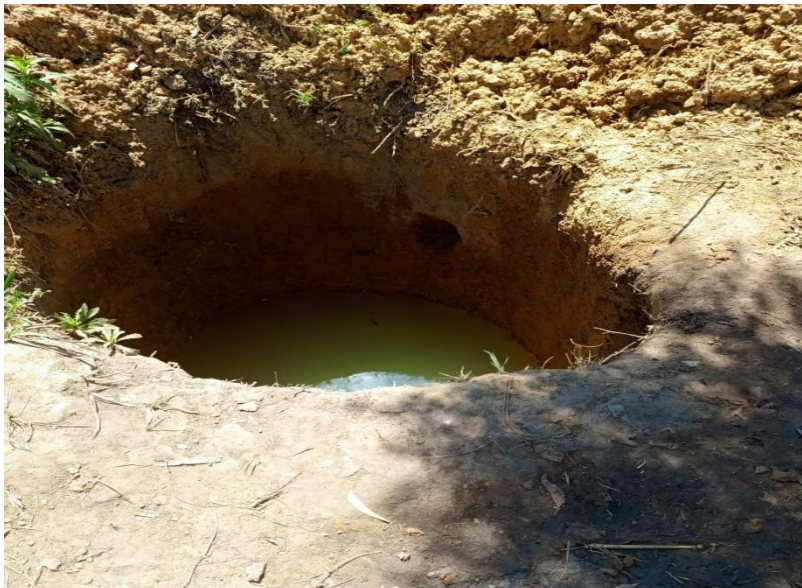
An unprotected well used for domestic water
