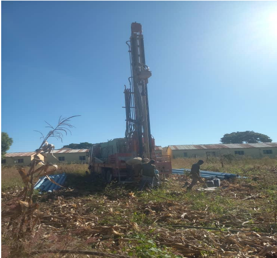
Photograph 4.53b: a borehole being drilled at a school to provide the community with clean safe water and to aid with irrigation water.
