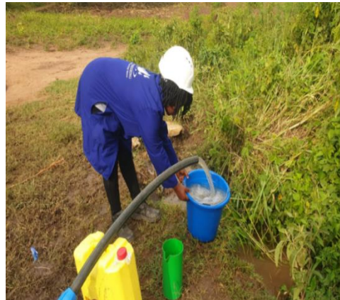
Figure 2:5 Borehole capacity testing (source: Mimishacirrigation.online)
