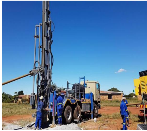
Figure 2:4 Borehole drilling (source: globaldrilling.co.zw)
