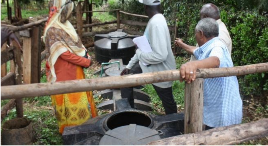
Picture 4 shows biogas digester buried underground.
