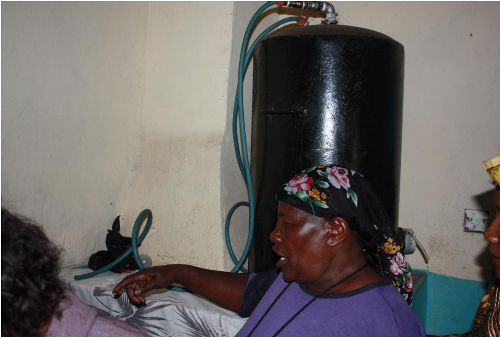
Picture 5 shows an ordinary LP gas cylinder modified to store the harvested biogas.
