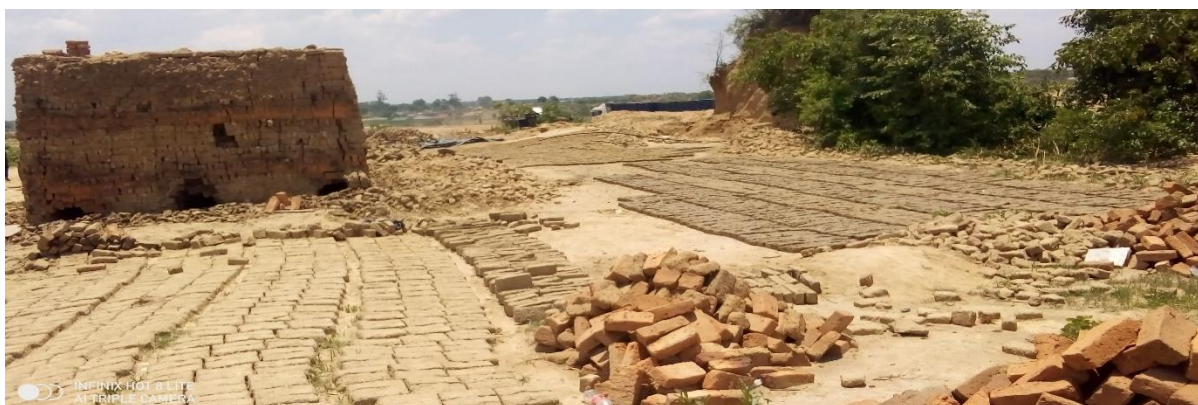
Figure 4.6: Brick moulding in progress
