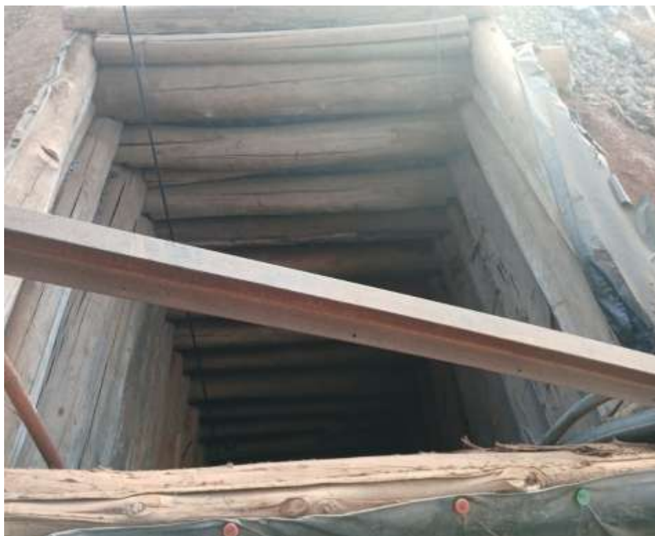
Fig 4.4 Timbering of a mining shaft
