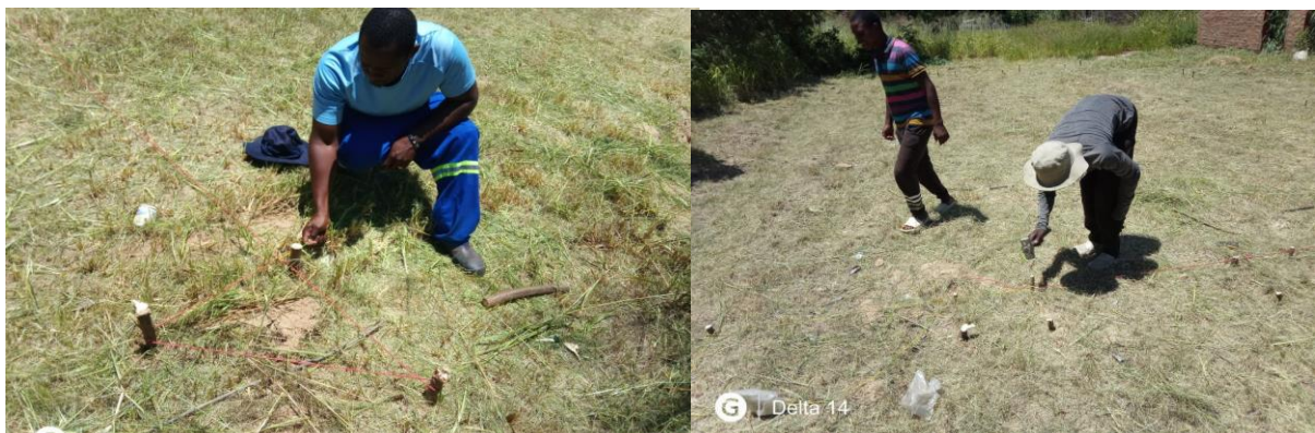
Figure 3.2 Pegging using the 3-4-5 Method
