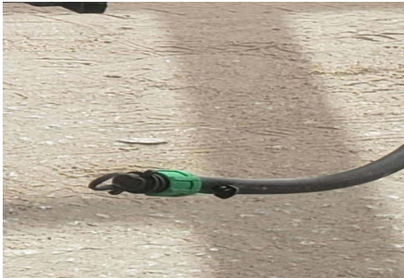
Figure 13: 0.5L/min nozzles and pipe
