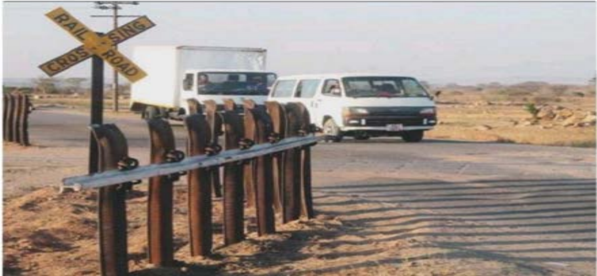
Figure 2.1 showing current railway-level crossing in Zimbabwe [1]
