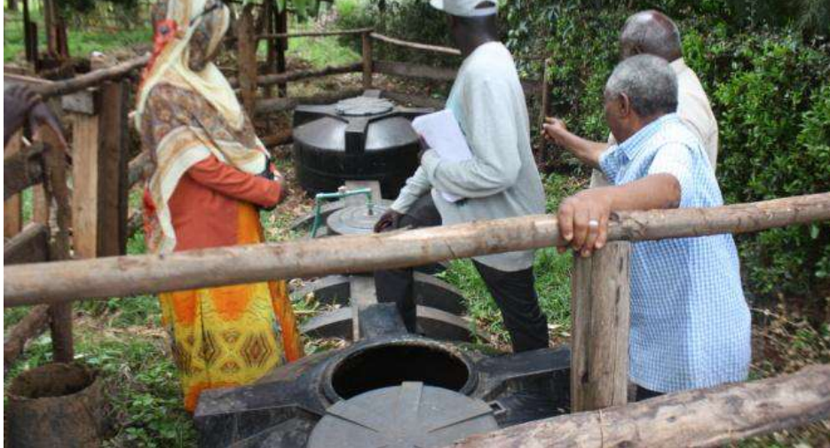
Picture 4 shows biogas digester buried underground.
