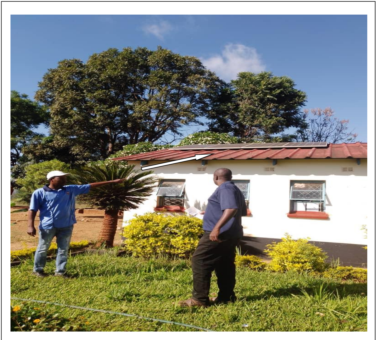
Image 1.2 highlights classroom block where a solar panel was stolen source field research 2024
