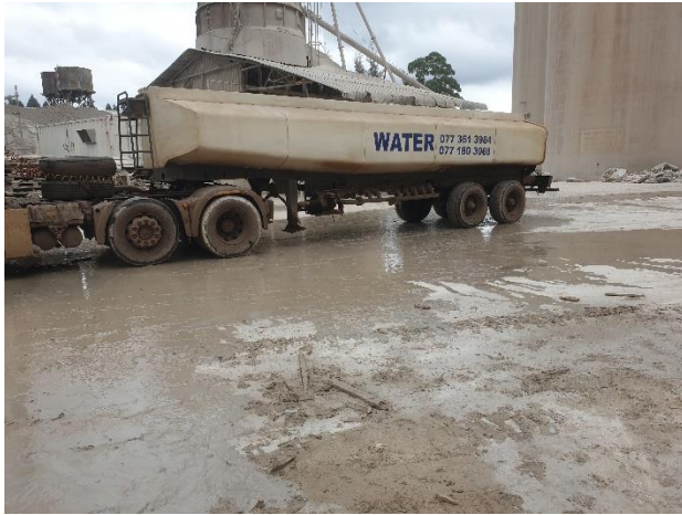
iii. Bulk water tank spraying water to suppress dust.
