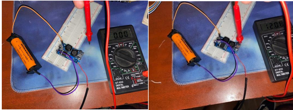
Figure 4.5: Image insert showing power supply implementation.
